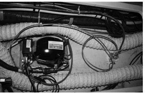
about \$100 more than the K35; however, for our modest size refer box (less than 7 cubic feet) the more efficient K35 seems more than adequate, especially since I was adding insulation to the fridge box. The smart speed controller option provides equipment protection and energy savings by automatically ramping up the compressor speed during start-up, and by adjusting speed during operation for optimum efficiency based on thermostat settings, ambient conditions, and load.
